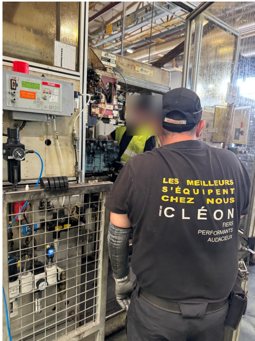
Image 8. The leak-tightness test bench (ATEQ F510/01 unit, on the left) at the time of the incident.
