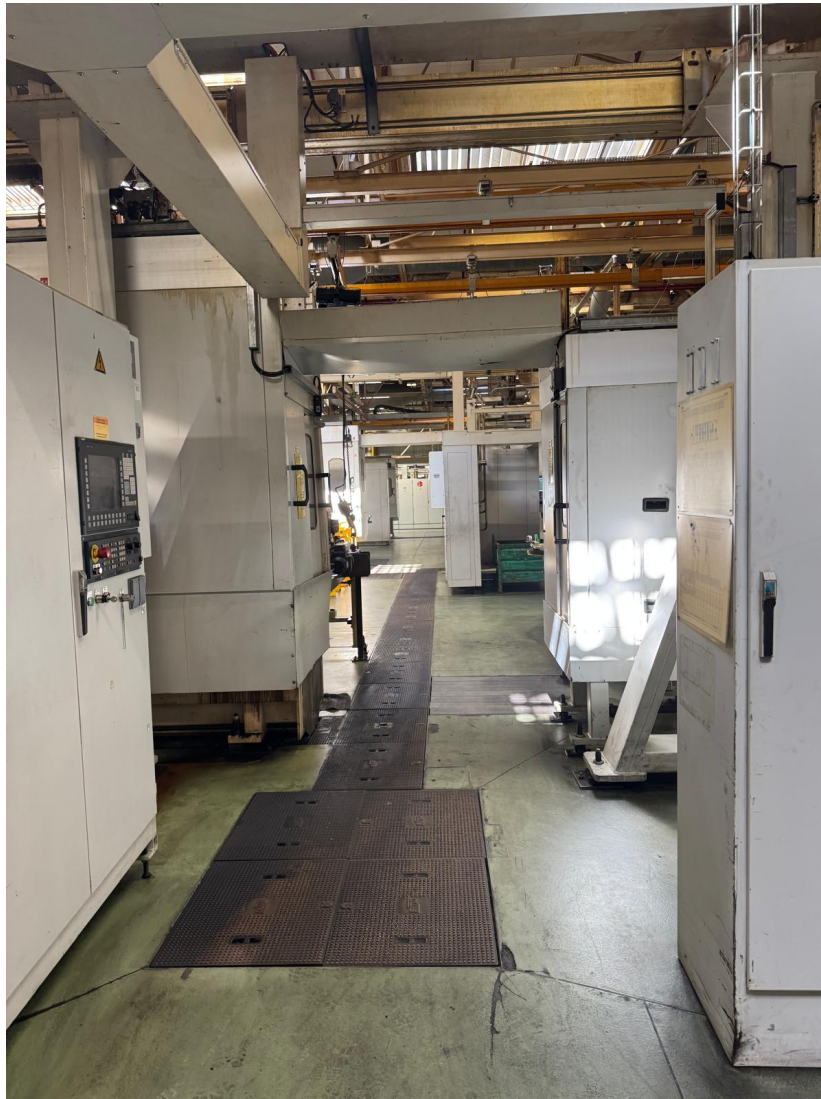
Image 22. Another aisle of the workshop, with its control panels and overhead cranes.
